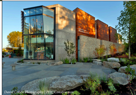
David Cohen Photography | PHC Construction
